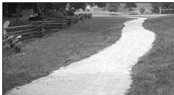
The finished pathways are more solid and easy to navigate through the museums at the park.
